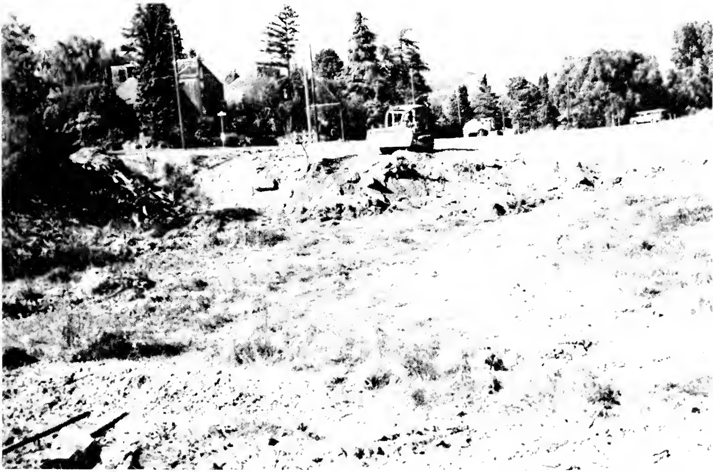
Bulldozing of the Conifer Meadow site. Photo: J.A. Witt
